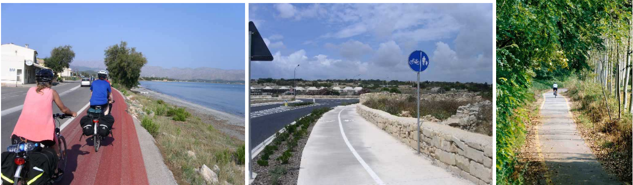
1. Cycle Lane Mallorca (Alcudia –Pollenca). 2. Cycle Track Malta, Halfar Road. 3. Cycle Track in separate layout. Lodi in Italy.
